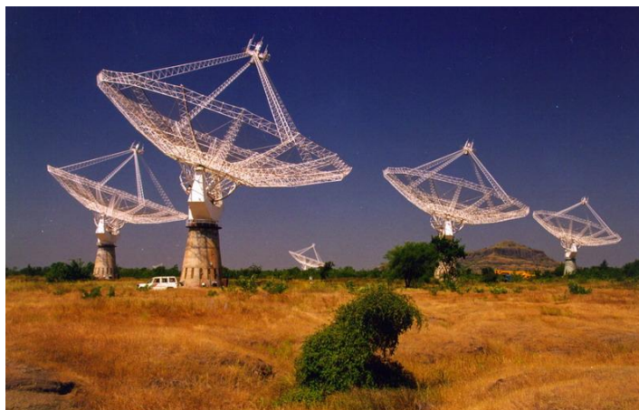
Fig-6: GMRT Antennas at daylight (Source: Official website of the GMRT)
